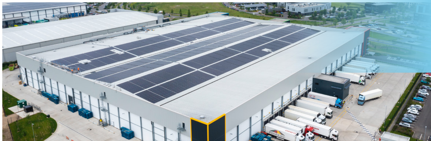
Large solar array at a warehouse in Huntingdon
