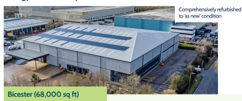
At Bicester, the warehouse was comprehensively refurbished, with the roof replaced, roof lights added and solar PV installed. We also upgraded the internal lighting and systems, replaced gas with a 47kWp electrical heating system and installed three EV charging points. The works have increased the EPC rating to 'A+' from 'C' and the 160kWp solar PV system is expected to save 28tCO<sub>7</sub>e p.a.
