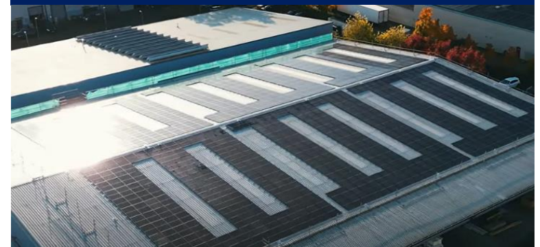
300kwp Solar PV & Battery storage at Bicester
